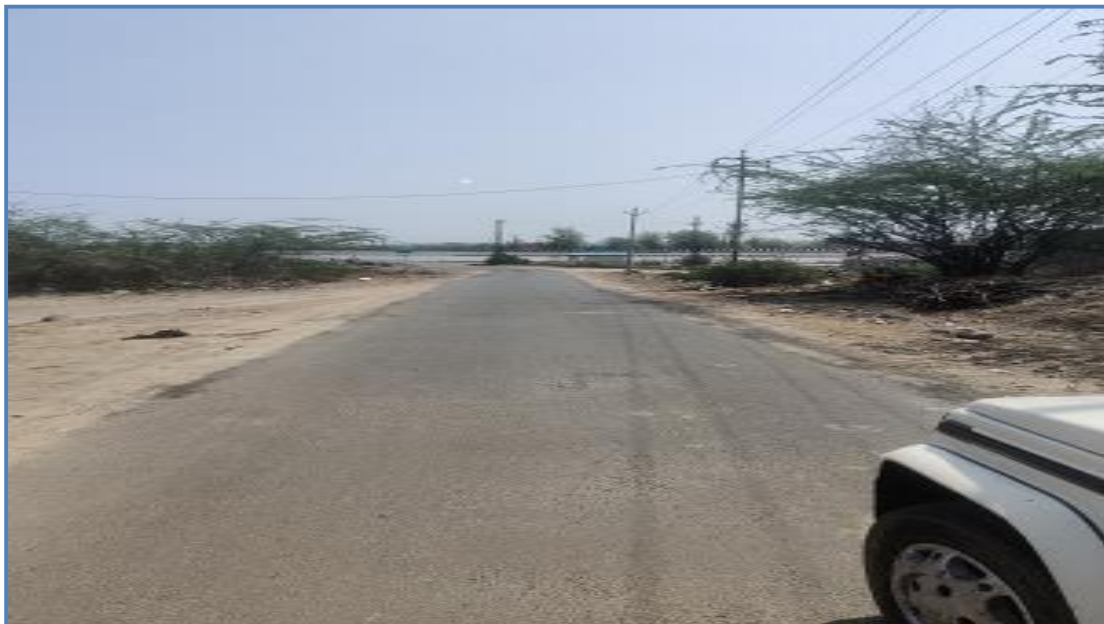
PHOTOGRAPHS OF RELAID BITUMINOUS ROAD OF HATHI BHATA CONNECTING TO NH-79
