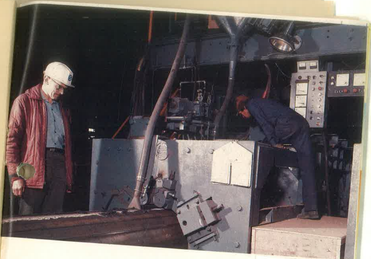
External Dia Welding
